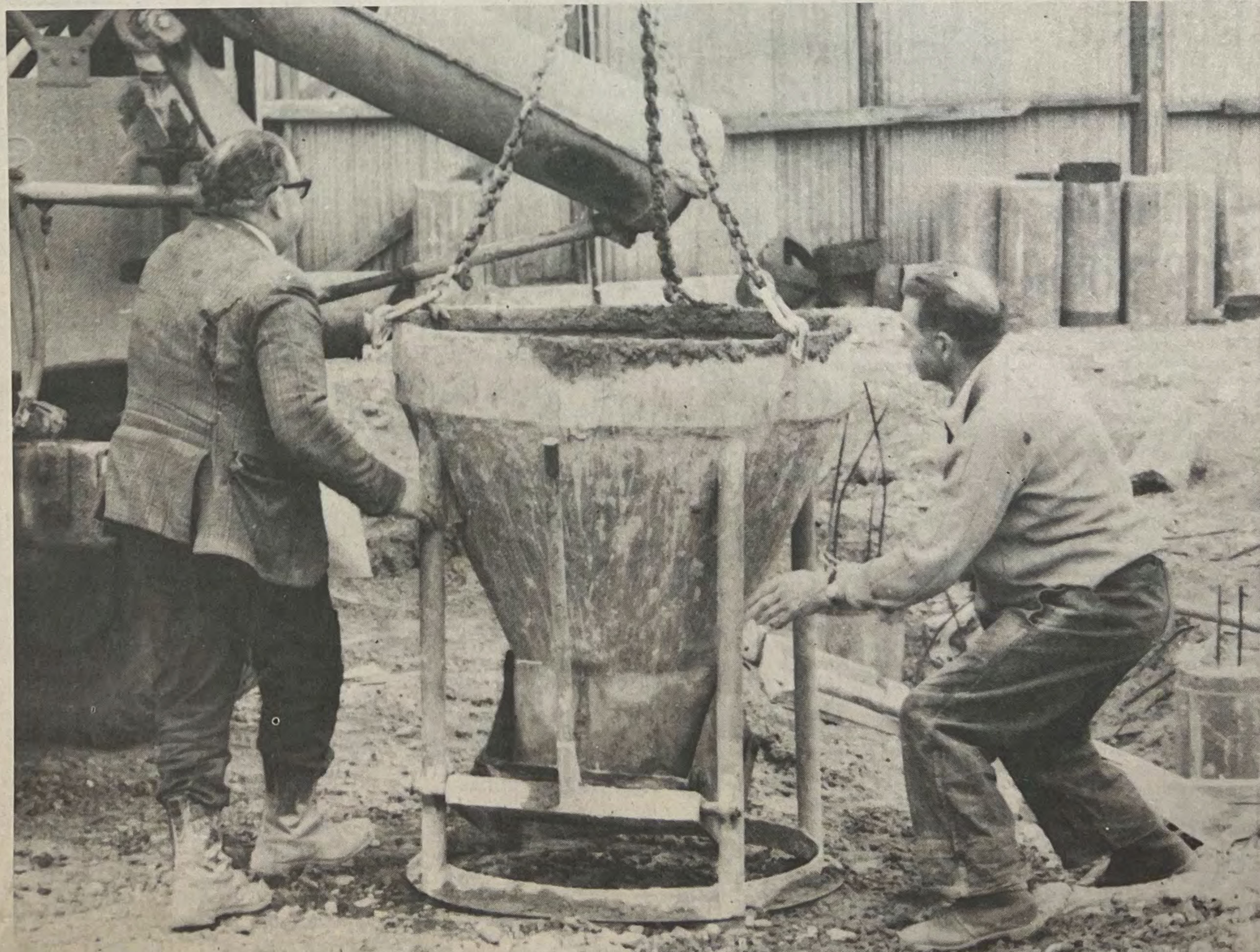
Hard at work on a Dublin site. No lumping here.
